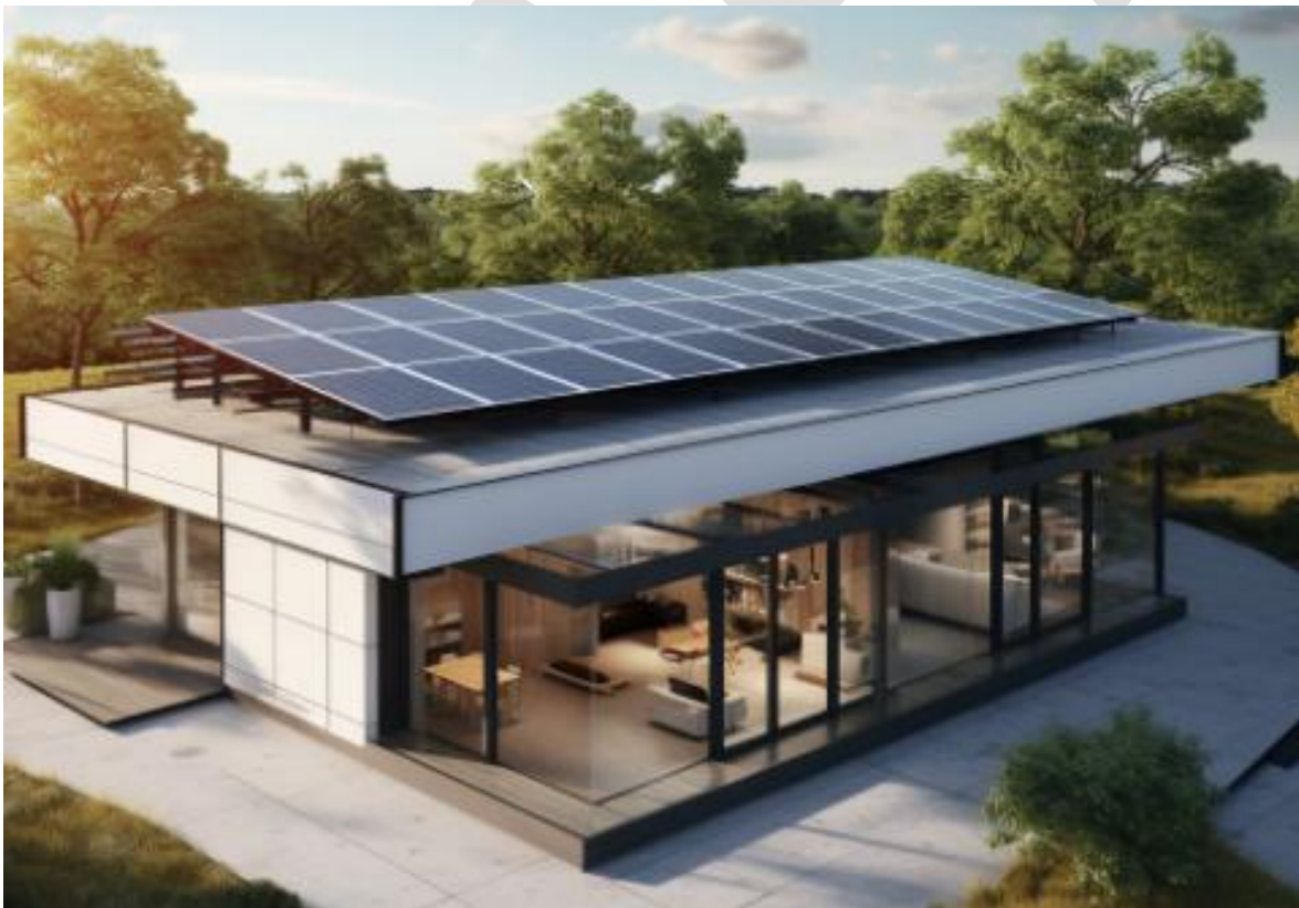
Panels on a flat roof without a parapet, mounted in an organized pattern, parallel-aligned with the edges of the roof.
