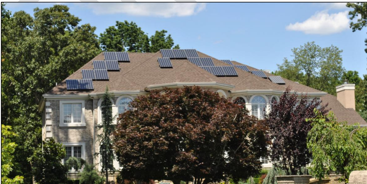
A disjointed arrangement of panels, on multiple roofs some configured in a stair-step pattern.
