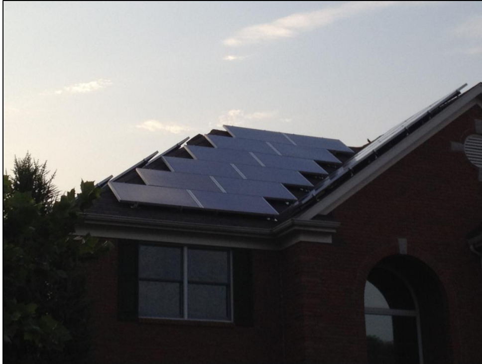
Panels configured in a stair-step pattern.
