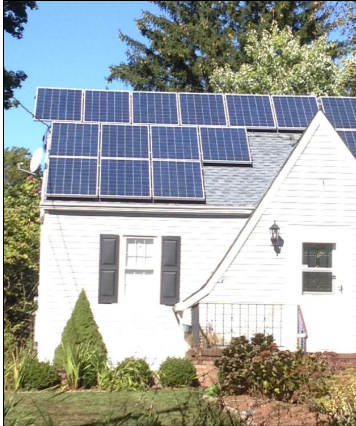
Panels extend to the edge of the roof and beyond.
